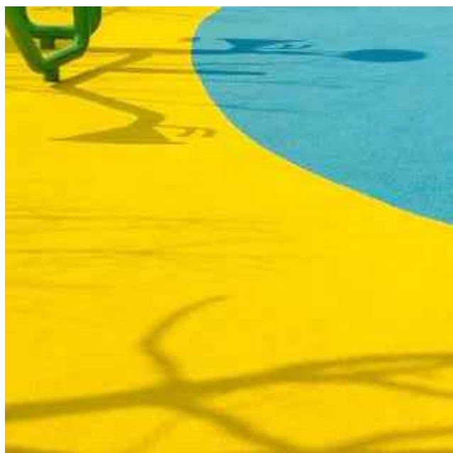
SOFT POUR SURFACE 15mm coloured epdm rubber crumb layer colours: tbd SBR layer base layer depth in accordance with standard requirements regarding critical fall heights Granular sub-base refer to engineer's specifications
