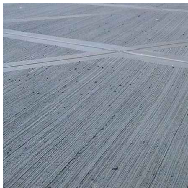
IN-SITU CONCRETE PATH In-situ concrete path 100-150mm concrete with polypropylene fibre reinforcement refer to engineer's specifications 100-150mm granular sub base refer to engineer's specifications
