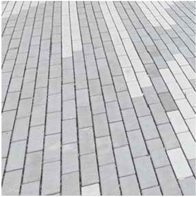
HIGH QUALITY PAVING 2 To public open space Type: Natural Stone Block Colour : Grey or similar approved Sub-base to engineer's design detail & specification
