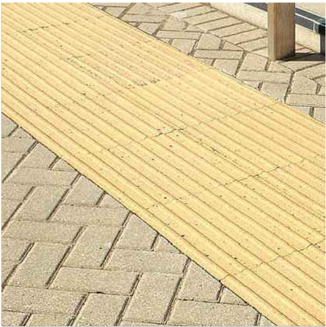
TACTILE CORDUROY PAVING TO TOP + BOTTOM OF STEPS 50(D)mm rapid set bedding mortar Granular Sub-base
