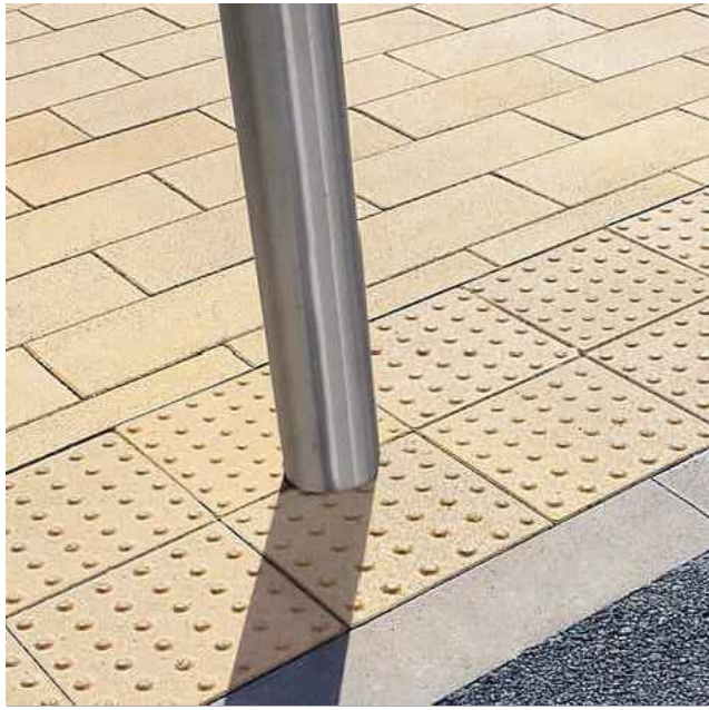
TACTILE BLISTER PAVING TO CROSSING POINTS 50(D)mm rapid set bedding mortar Granular Sub-base
