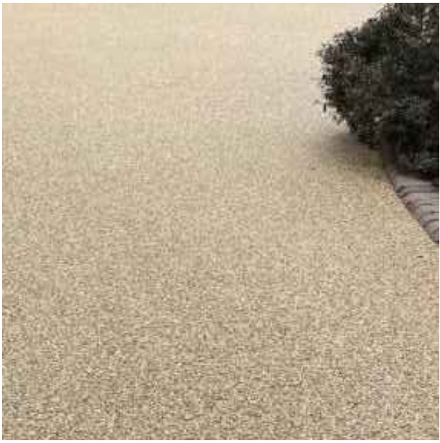
COLOUR FINISHED SMA TO RAISED TABLE & SHARED SURFACE Colour : TBD or similar approved Asphalt refer to engineer's specifications Sub-base to engineer's design detail & specification
